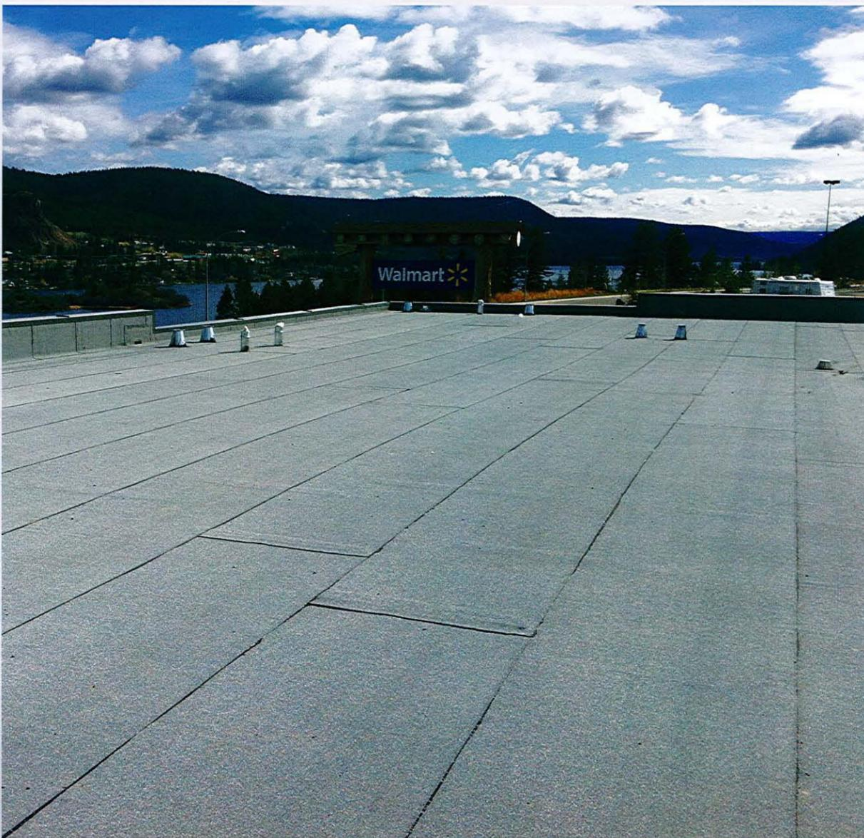
Mainline installed "bullet proof" 2-ply SBS on the roof of the Prosperity Ridge Shopping Centre in Williams Lake. Photos: Mainline Roofing
